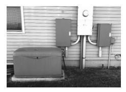
power goes out. They run on propane or natural gas and cost \$3,000 to \$6,000, not including installation. Do not try to install a standby generator on your own; they should be installed by an experienced electrician.
